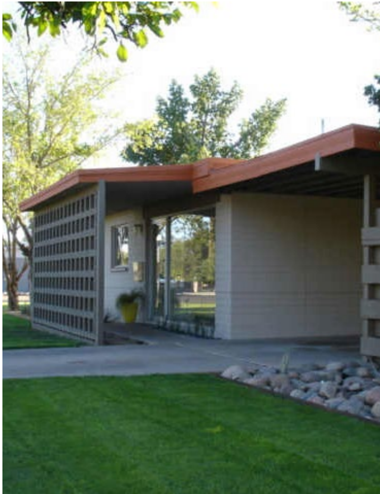
Front Entrance Daksiewicz PHX Residence
